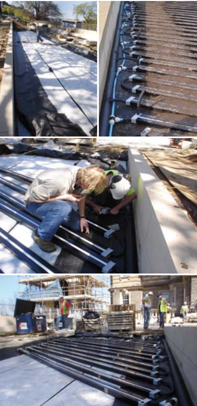
Fitting Tanker Modular network up to 4m long with full automation to restricted depth roof garden for fine turf
