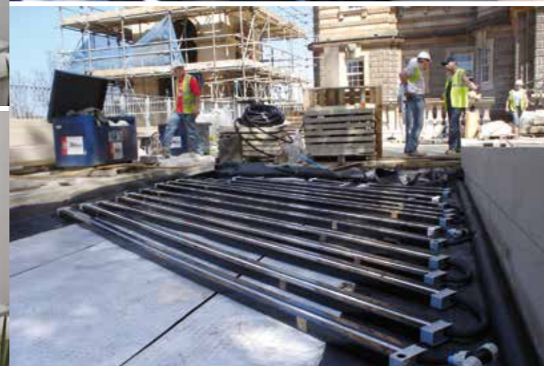
Fitting Tanker Modular network up to 4m long with full automation to restricted depth roof garden for fine turf
